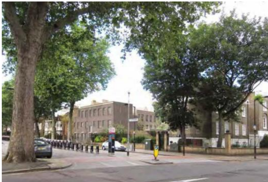
View of Block E from the junction of Braganza Street and Doddington Grove
